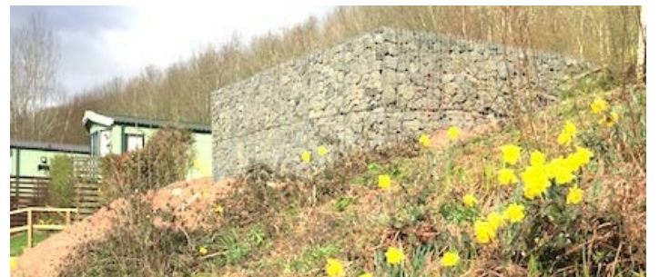
The new gabion wall ready for the Victory Lodge
